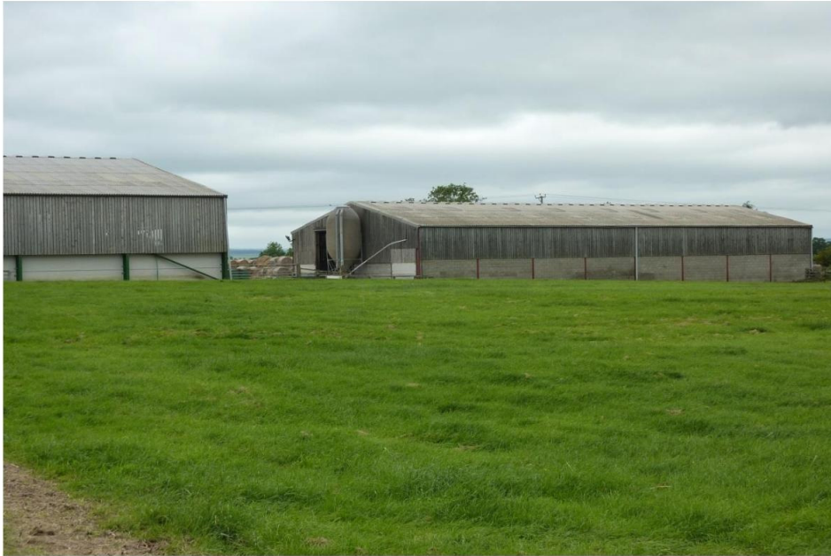
Photograph 1- View of existing farm buildings along southern boundary of farm yard
